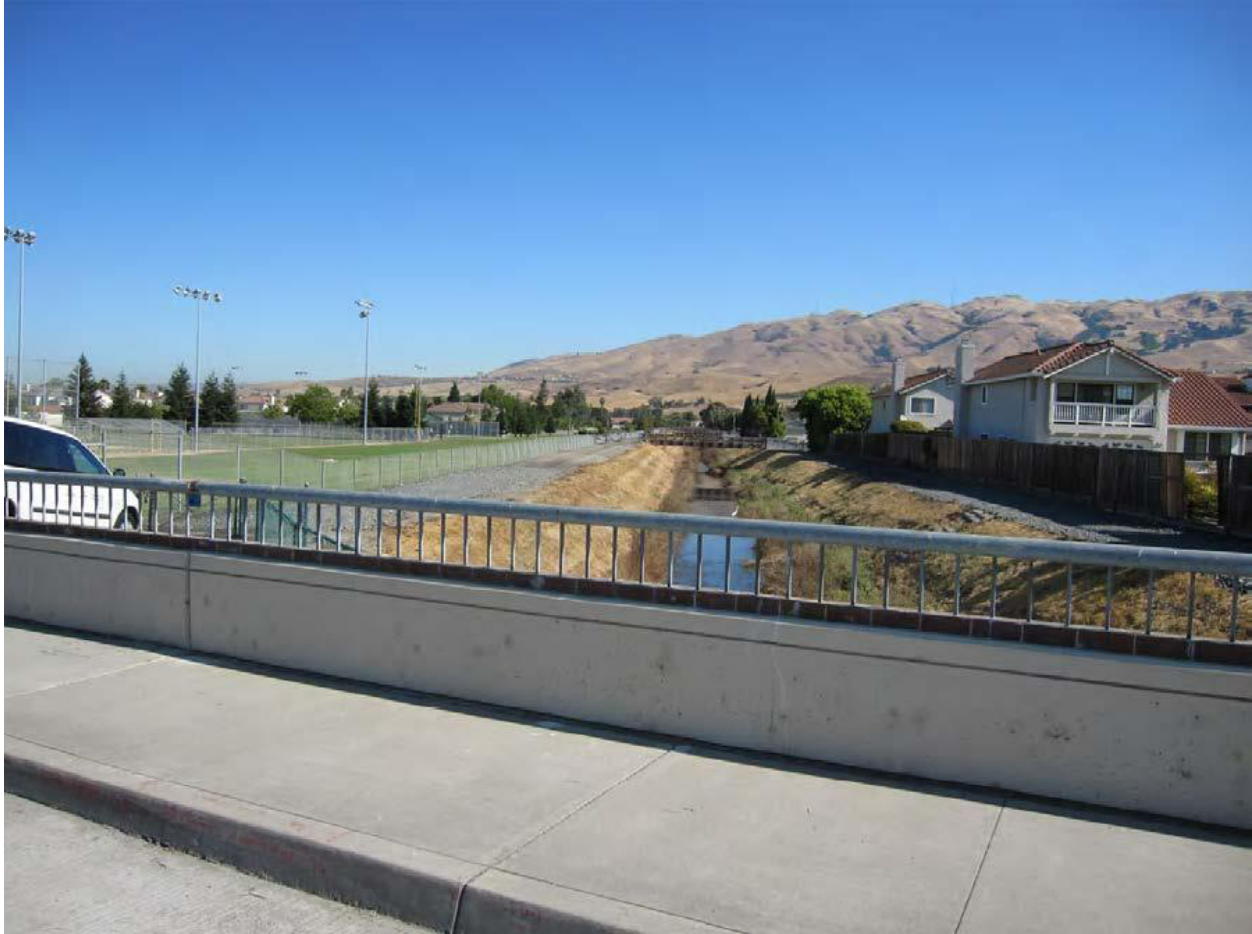
Figure 3-2 North View of Tularcitos Creek (looking upstream) from Paseo Refugio
